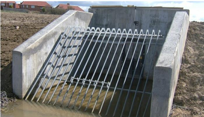
Culvert Grille with Access Hatch
