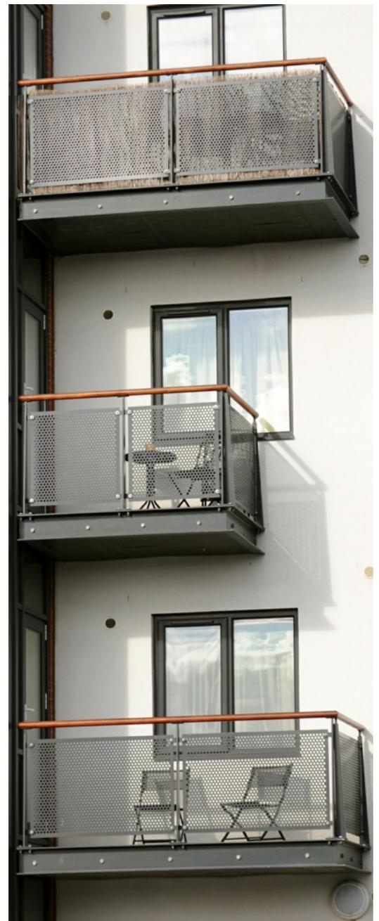
Perforated Plate & Timber Rail Balconies -
