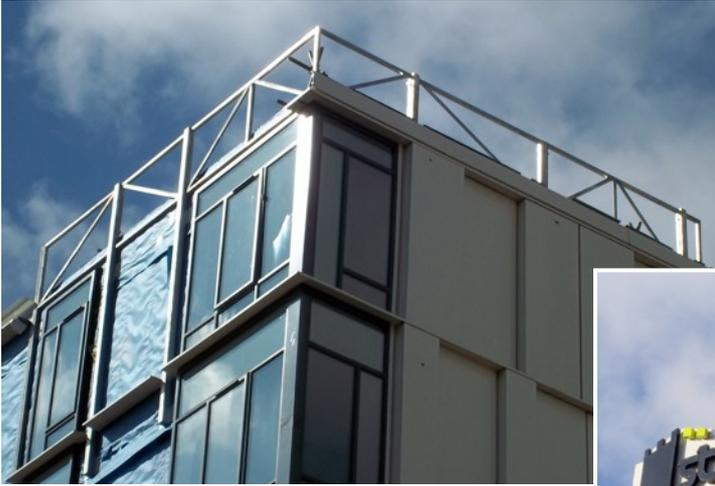
Steelcraft has fabricated and installed a range of secondary steelwork items which are inevitably made-to-measure to suit specific applications.
