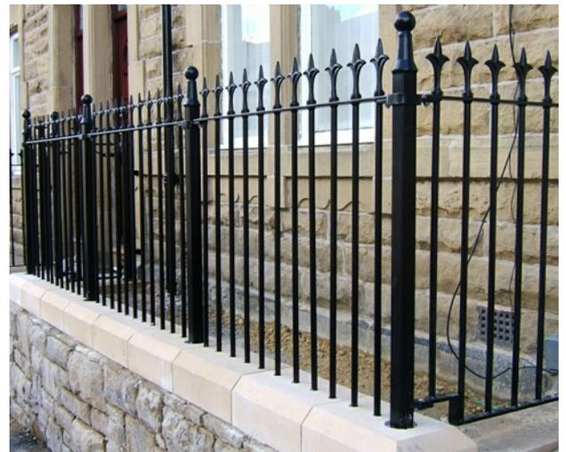
Railing with Each Vertical into Coping - Housing Regen in Gateshead
