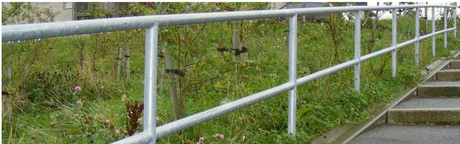
Tubular balustrade is generally used externally to offer support for pedestrians using stairs, ramps or pathways. It is also used to protect the public from hazards.
