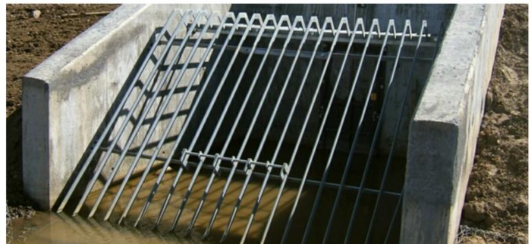
Culvert Grille with Access Hatch
