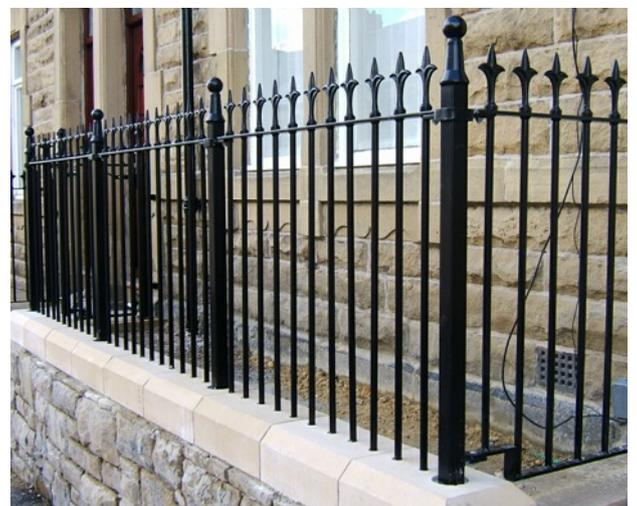
Railing with each Vertical into Coping - Housing Regen in Gateshead
